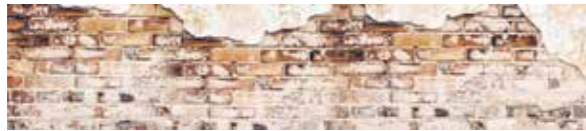
323 Ziegelwand 323 Brick wall
