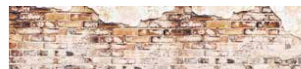
323 Ziegelwand 323 Brick wall
